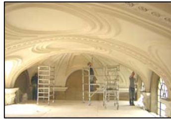
Distemping of the ceiling
