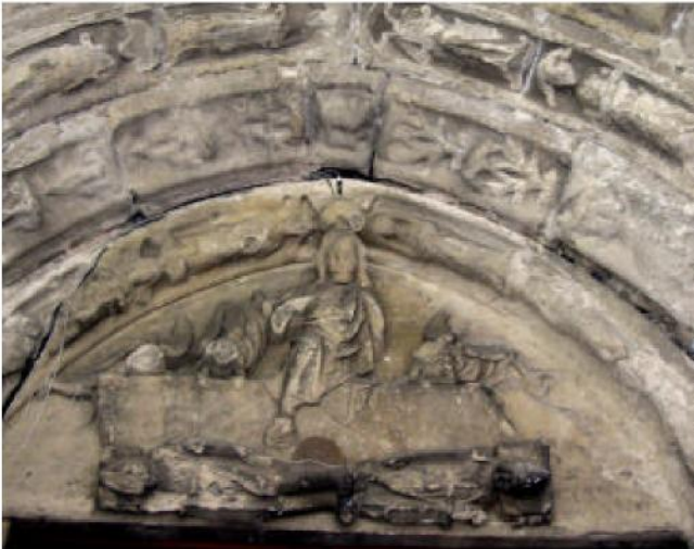
Destroyed Romanic portal
